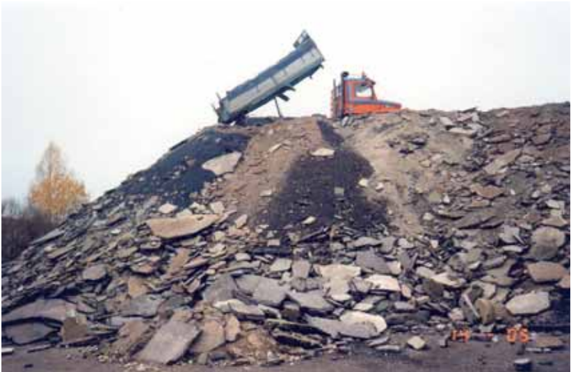
Unloading sheets of asphalt concrete
