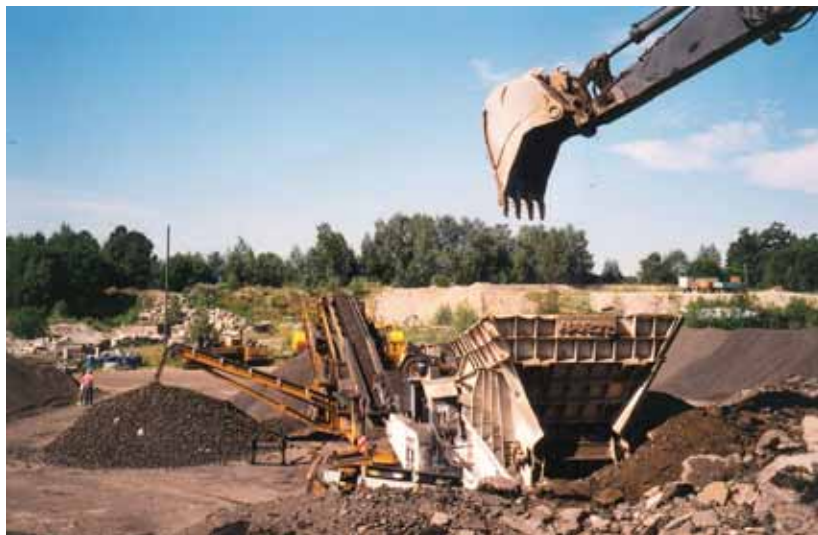
Crushing and sieving of reclaimed asphalt
