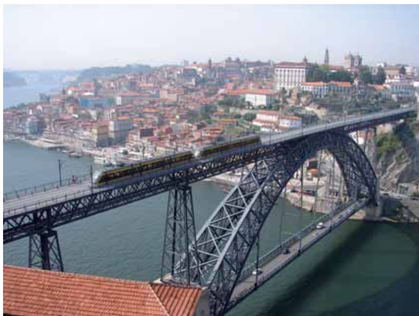
Metro over Douro river in Porto, Portugal
