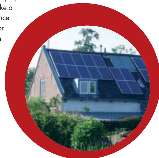
Roofing products installed in an amateurish way
