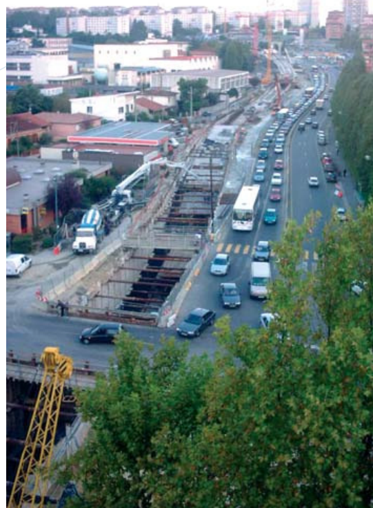
General view of a cut and cover project in Toulouse, France
