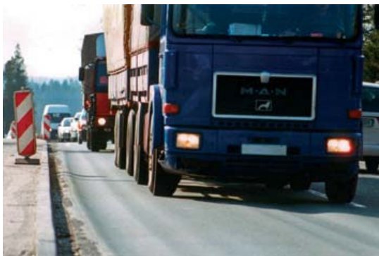
Example of an under-designed pavement
